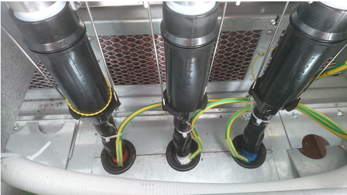
**Figure 11 – Transformer cables in tee-off endbox**
