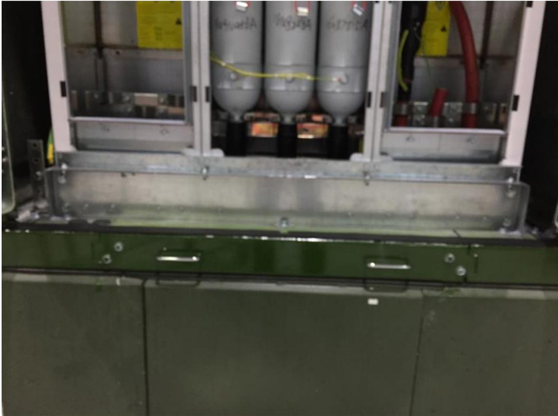
**Figure 6 – Lower part of the RM6 RMI with endbox covers removed**
