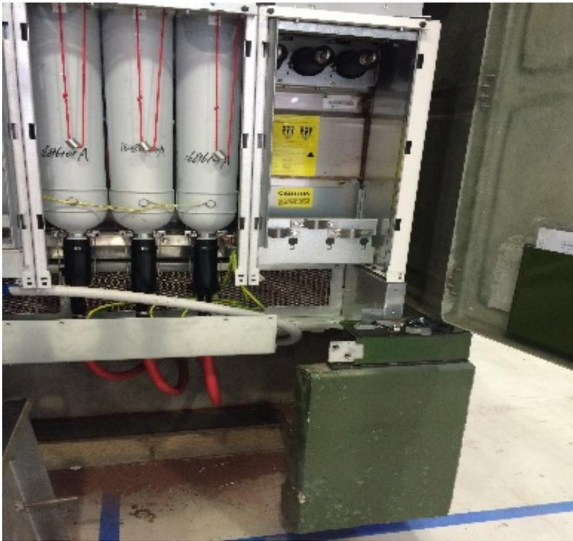
**Figure 15 – Cable installation with full access**
