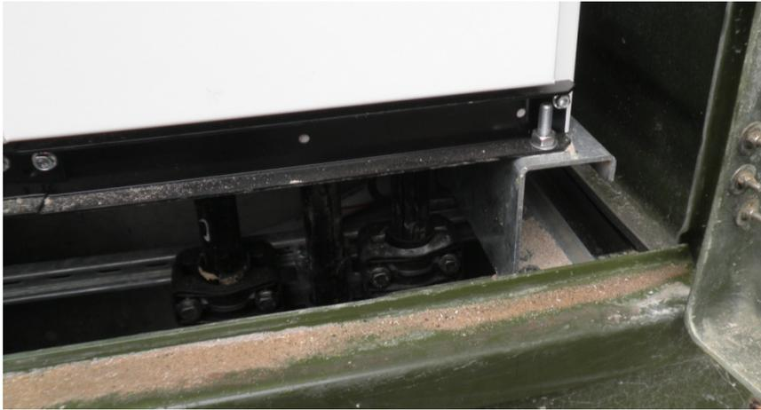
**Figure 12 – Existing cable cleat bar now replaced by internal endbox bracket and supports**
