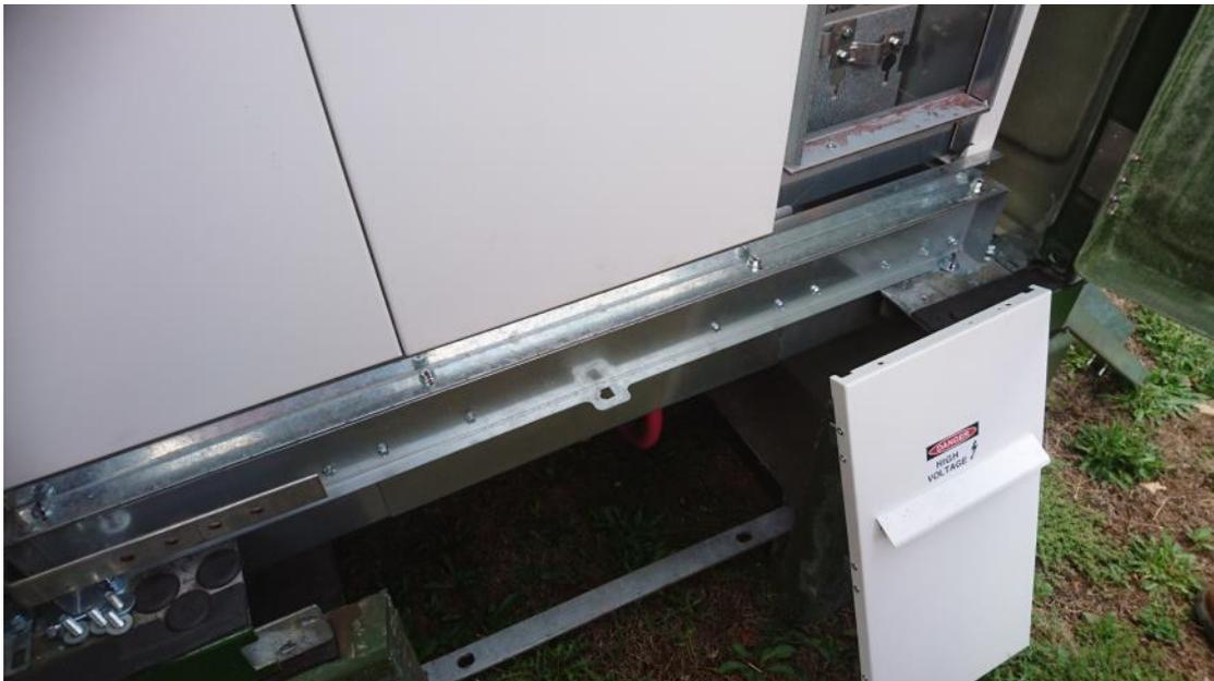
**Figure 7 – Top lintel (Fibreglass), D-pull handle lintel, Concrete base access cover (lintel) and RHS endbox cover removed**
